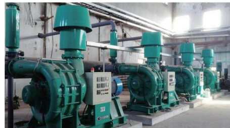
大庆肇源污水处理厂 Zhaoyuan Daqing sewage treatment plant
